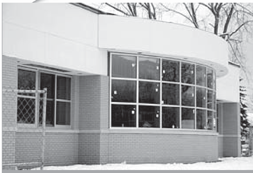
An exterior view of the new Saddlewood Elementary School library addition.
